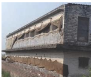
Use of gunny bags for prevention of cold air entering in shed
