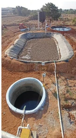
Primary Digester & Pumping Tank
